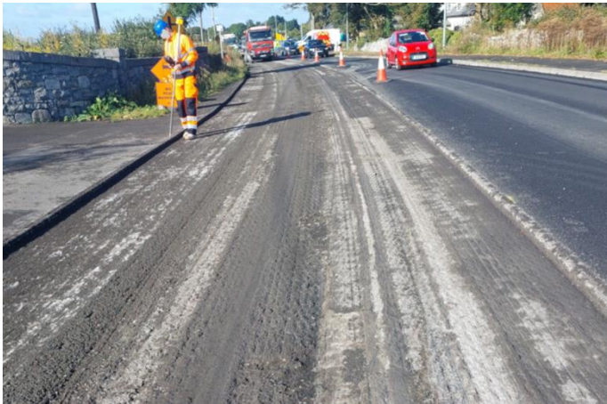
COAST ROAD FOOTPATH AND ROADWORKS
