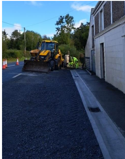
SMALL NOM FUNDED DRAINAGE AND CHANNEL KERBING PROJECT AT CASTLEDALY
