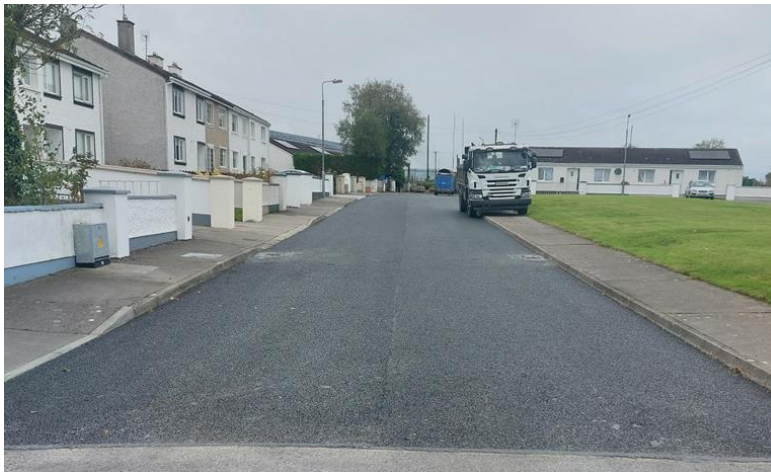
ROAD RESURFACING - CLOUGHBRACK HOUSING ESTATE, EYRECOURT
