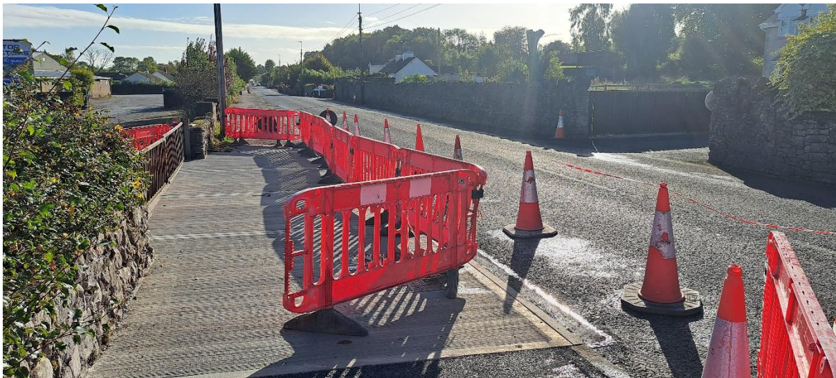
FOOTPATH REPAIRS AT MART ENTRANCES – CLEAGHMORE, BALLINASLOE
