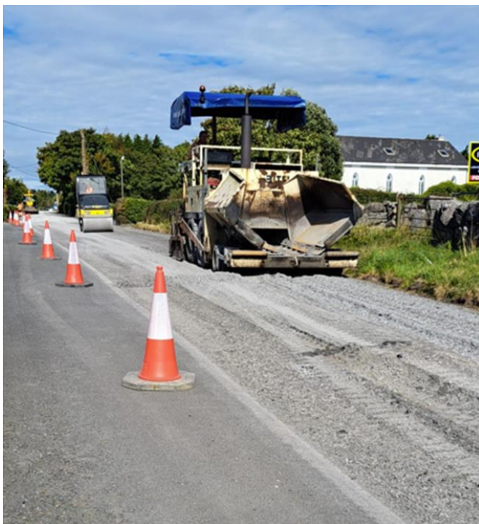
L-8580 – ROAD RECONSTRUCTION WORKS AT DUNKELLIN
