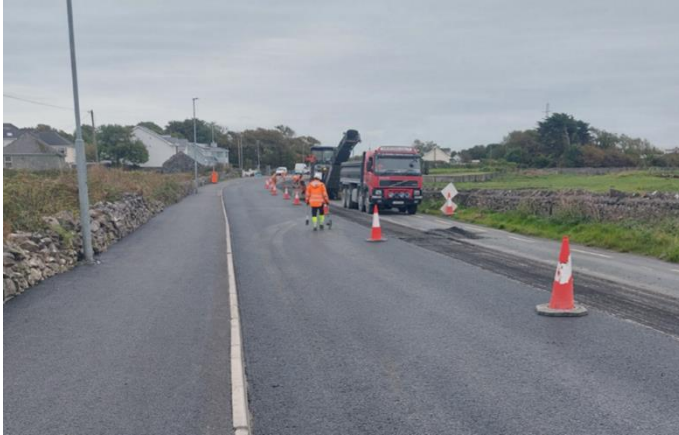
COAST ROAD FOOTPATH AND ROADWORKS
