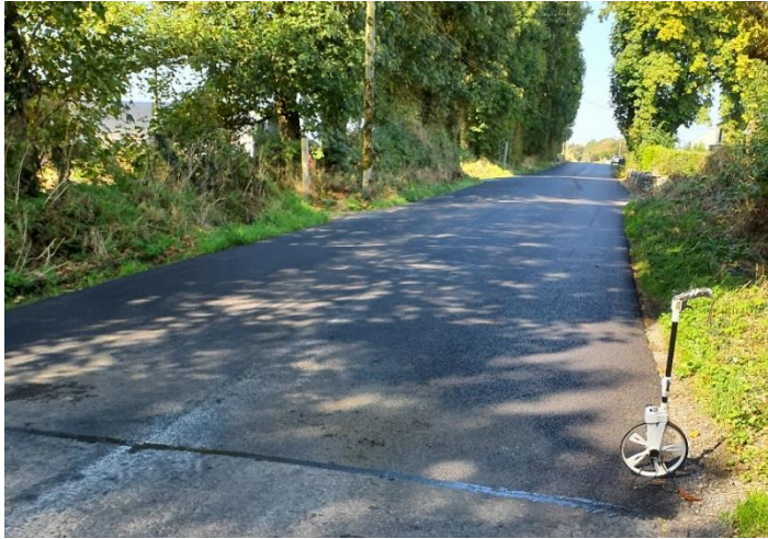
RI GRANT WORKS NEARING COMPLETION AT BALLYEDMOND
