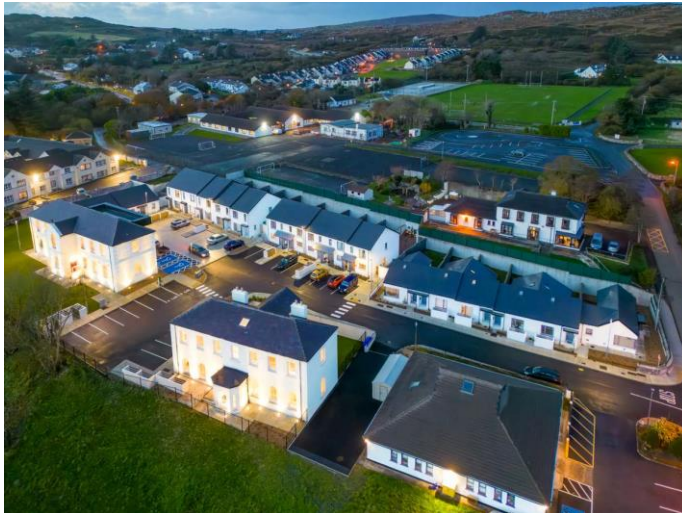
GORT NA GCLOCH, CLIFDEN – AN AERIAL VIEW OF THE COMPLETED DEVELOPMENT
