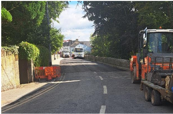
RI WORKS AT BRIDGE STREET, BALLINASLOE, WORKS UNDERWAY, AND COMPLETED (BELOW)
