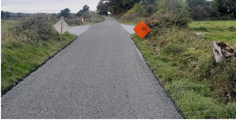
RI WORKS UNDERWAY AT POLLBOY, BALLINASLOE
